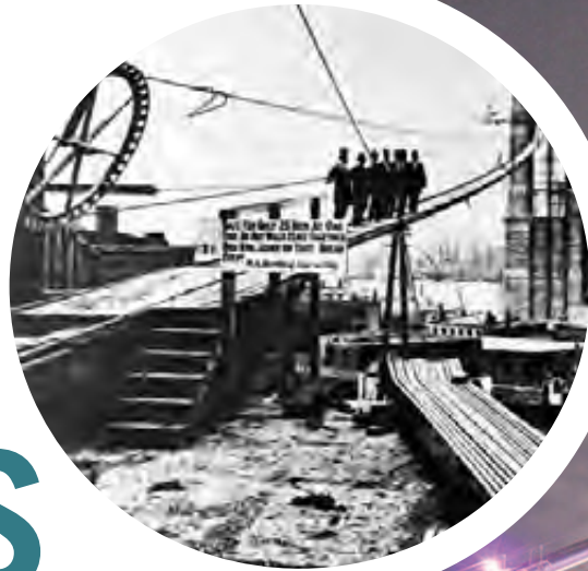
(right) Fig. 2: The John A. Roebling's Sons Company's innovative construction of the George Washington Bridge cables set the stage for its construction of the Golden Gate Bridge cables five years later.
