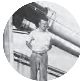
Fig. 10: Allen Searls on top of the Fort Lee Tower, with the cable wrapping nearly complete, 1931. Jan Searls and Doc Searls
