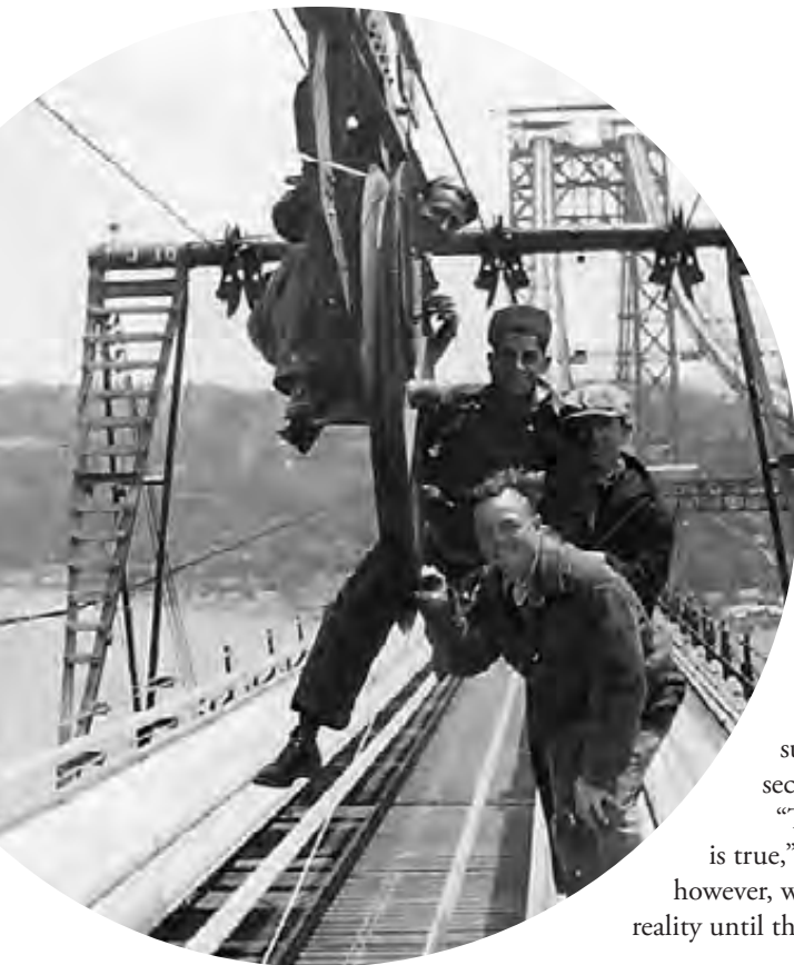
Fig 1: Allen Searls' photo of cable spinners with a Roebling Traveling Wheel on the George Washington Bridge, c1930. Jan Searls and Doc Searls.
