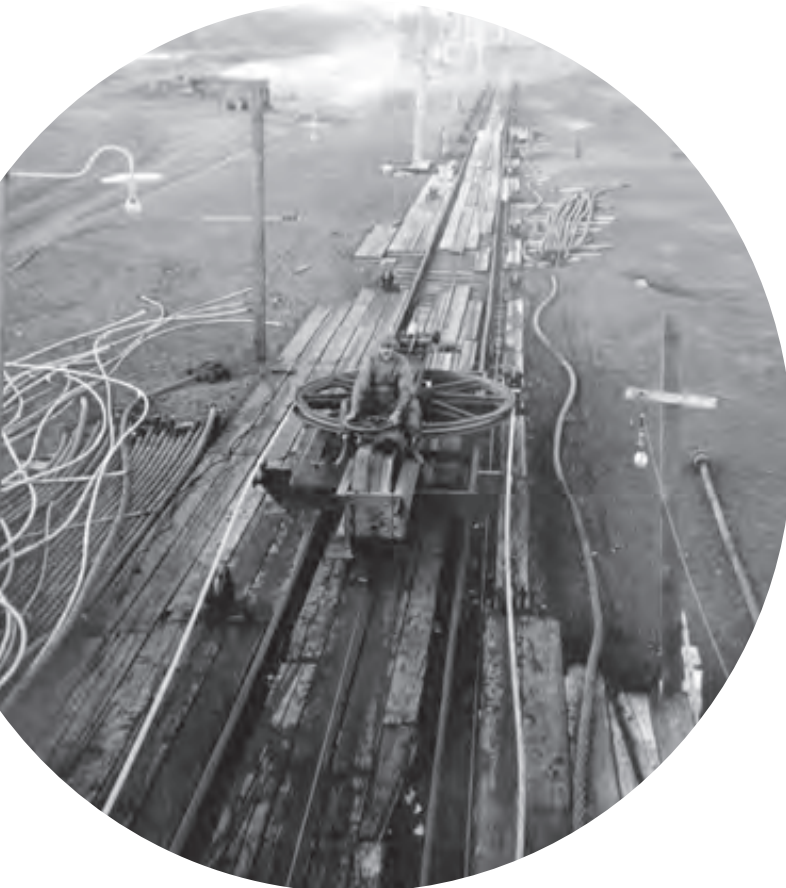
Fig. 8: John A. Roebling's Sons Company Prestretcher at the Kinkora Works, Roebing, N.J., c1929. The Company developed the innovative 1,850-foot long track to prestretch the footbridge ropes for the George Washington Bridge. Smithsonian Institution.
